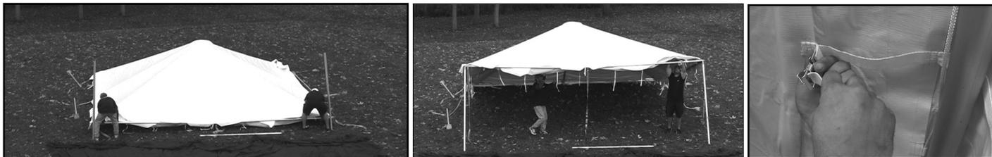
13. While the tent is still low to the ground fasten the rest of the alligator straps around the perimeter tubing.
