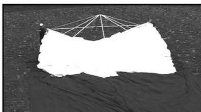
9. Loosely fasten 2 alligator straps at each corner around the perimeter tubing to secure the tent top.
