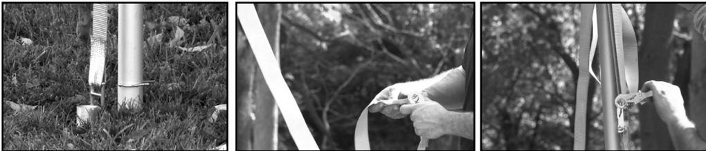
15. Repeat with the other side of the tent. When finished with the corner legs, install all other legs at side tee fitting locations. Pull the anchoring devices (ratchet buckle strap) through the tops of the hook and loop extensions on the tent top to provide access to the stakes.
