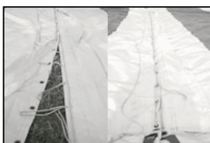
8. Pull the tent top over the frame, lifting up on the fabric or “flapping” it to create a cushion of air. Make sure the tent top is centered from all sides.
