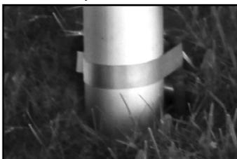
15. Roll excess ratchet straps and secure into the box ratchet buckle.
