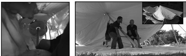
10. Tie off the jump rope attached to the center pole location (eye level: 5-6 feet).
