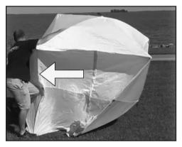
6. Once the entire frame is locked in place, stake the rest of the bottom-flap grommet locations or connect ropes to the metal eyebolts in the center of the walls and anchor the ropes to stabilize the shelter.
